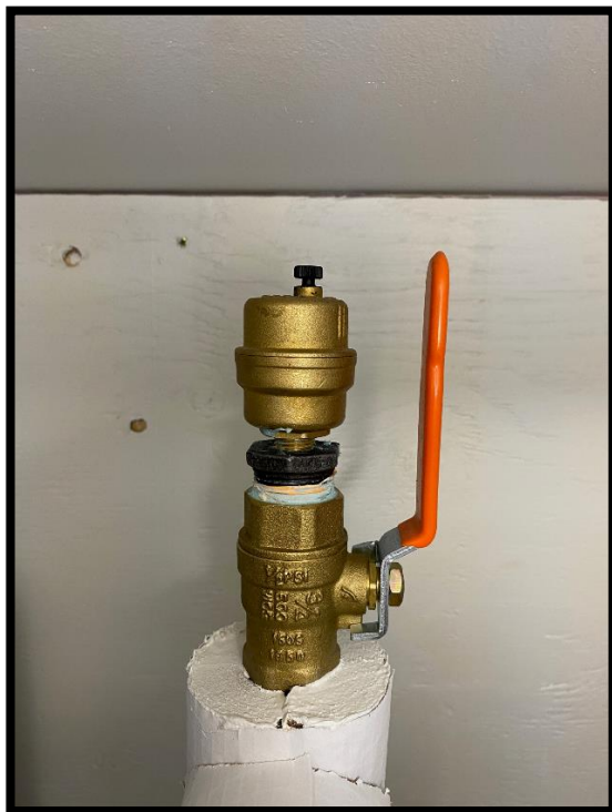
Caleffi 1/2" air vent and Ivar manifold with built in air vent.
