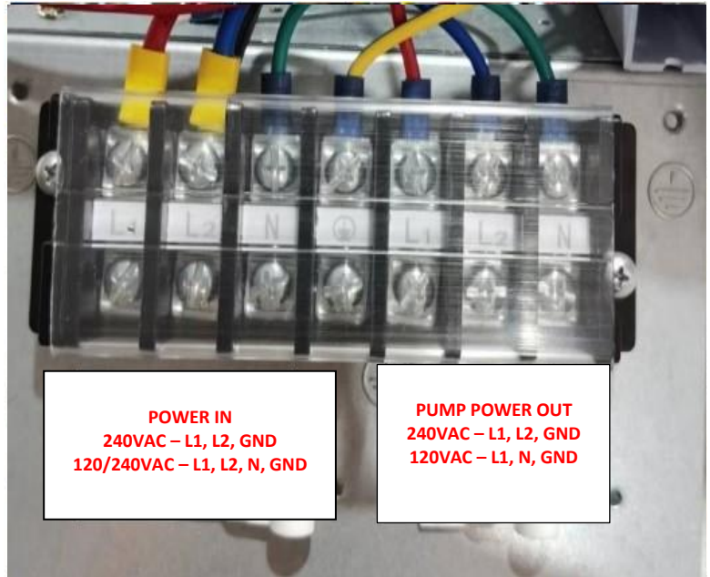
Connect Main & Pump Power
