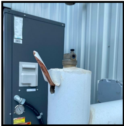
Typical air vent installation with insulation and shut off valve on the outlet line of the heat pump.
