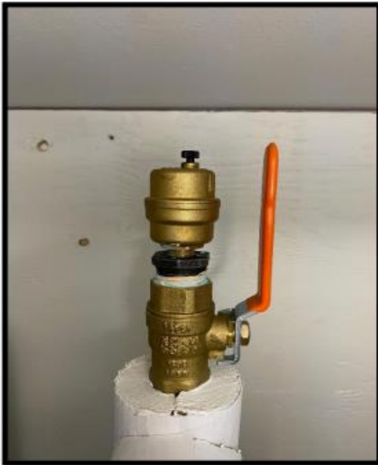
Caleffi 1/2" air vent and Ivar manifold with built in air vent
