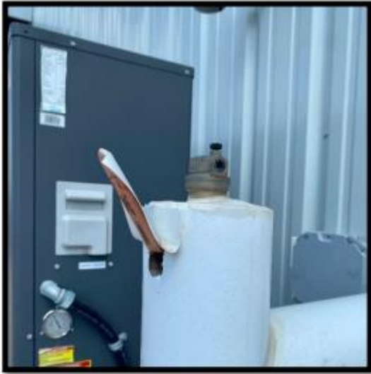
Typical air vent installation and shut off valve on the outlet line of the heat pump
